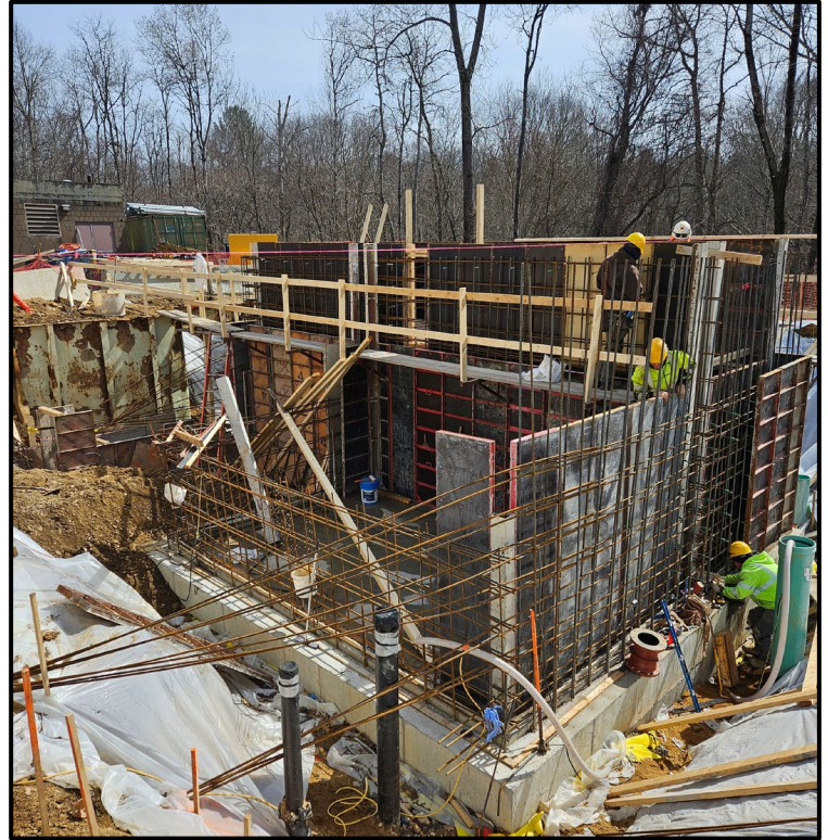
Installation of Rebar and Formwork for Effluent Clearwell Walls
