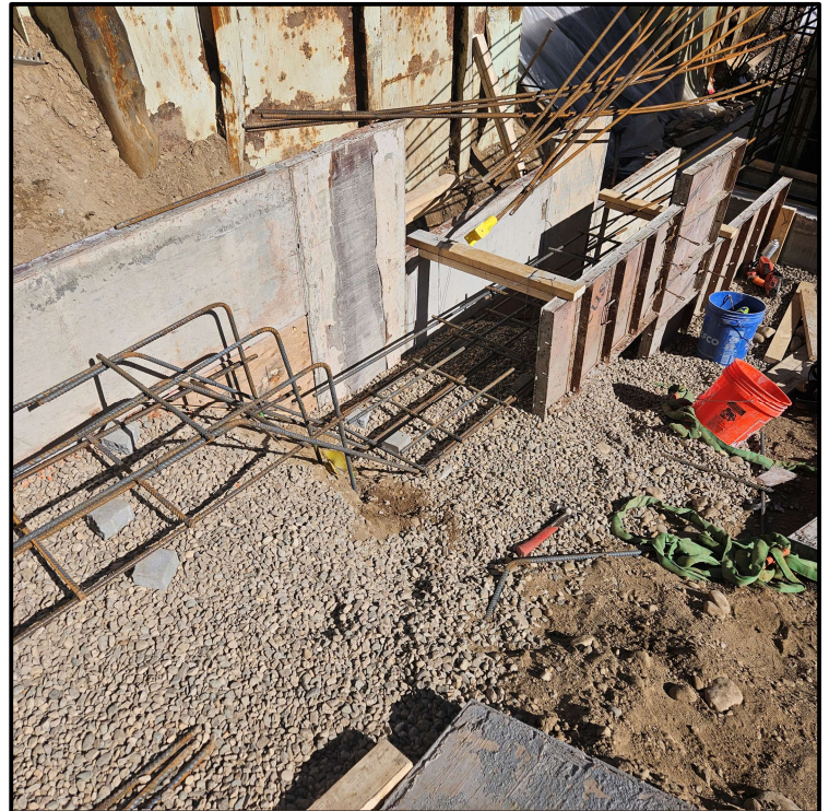
Installation of Rebar and Formwork for Stepped Footings of New Effluent Building
