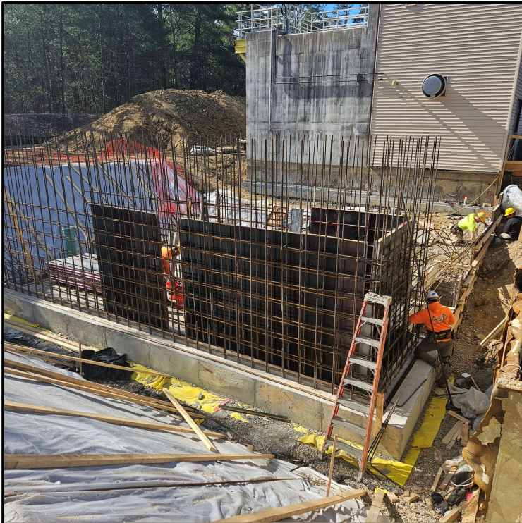
Installation of Rebar and Formwork for New Effluent Building Walls
