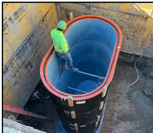
Installation of Wetwell/Valve Vault
