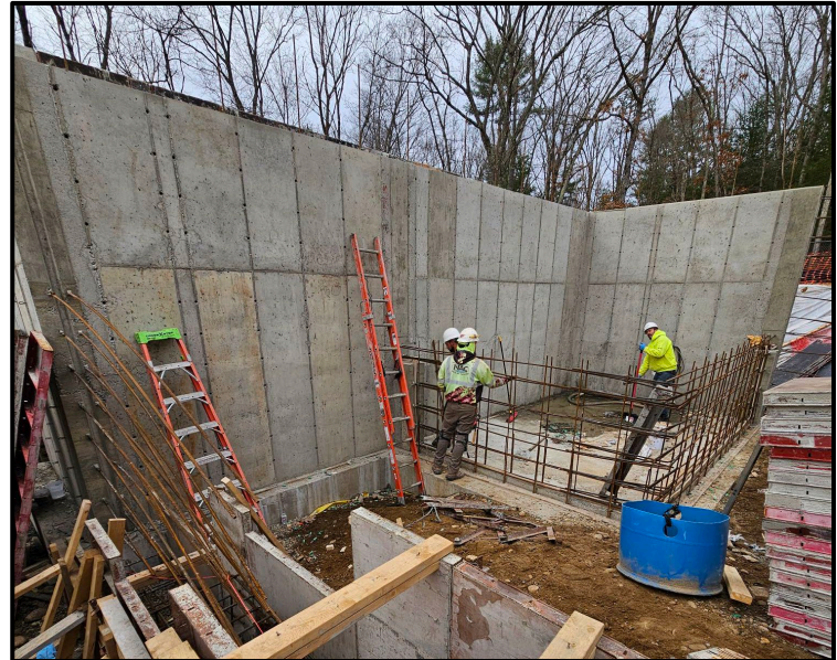
Effluent Building Rebar Installation
