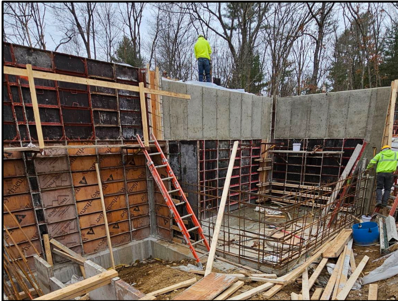
Removing Forms from Effluent Clearwell Walls
