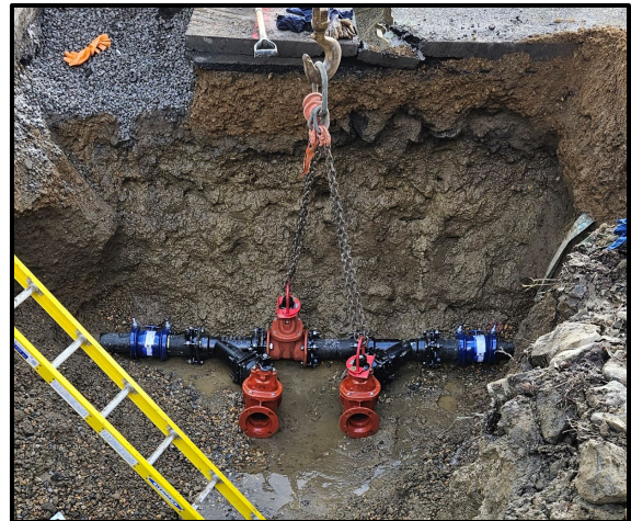
Placing Valves
