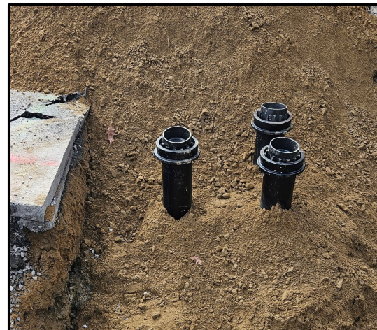
Backfilled Trench
